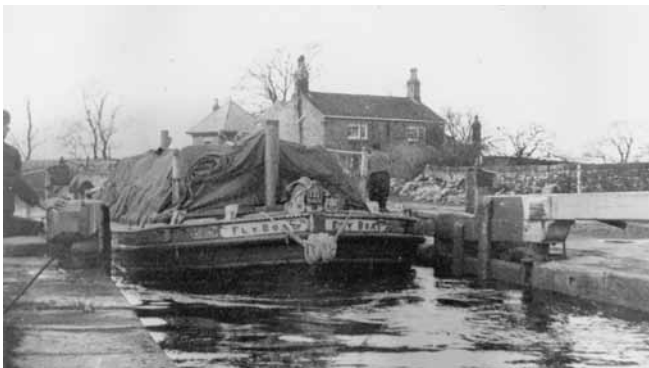
A flyboat entering Greenberfield top lock around 1900. Note the 'knighthead' above the stem post, a reminder that L&LC boats originated from coastal sailing craft. Note also the bar under the left-hand balance beam used for holding the gate open or closed.
