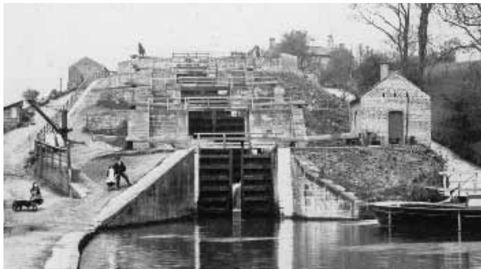
Bingley c1900. Note that balance beams were painted white with a black, curved-sided strip.
