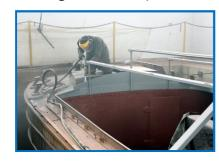
We have replaced the hold superstructure with new steel work, lutchet and roof boards to give a more traditional look. Work is now almost complete on the repainting of the topside and signwriting, in the livery of Canal Transport Ltd, Liverpool which will give Kennet her own new identity. After the new sheets have been fitted, Kennet will come out of Snaygill Boat's New Wide Beam Dry Dock on **Monday 21st May – a day** for your diary – come and have a look.
